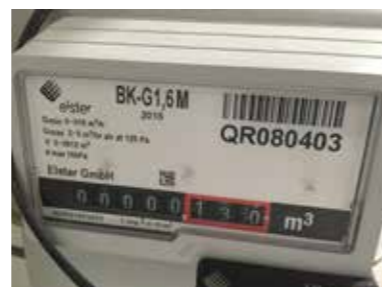
Figure 10.6b: Hot Water Meter
